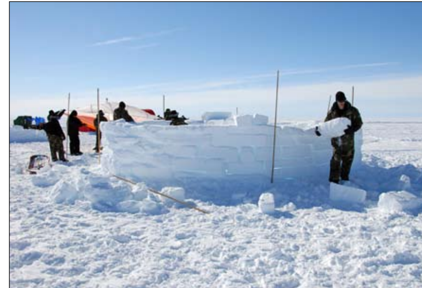
"Kool School" members construct a paradome. The snow structure is a shelter to help keep people warm from the cold weather.
