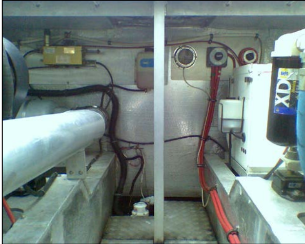
(Engine compartment view aft)
