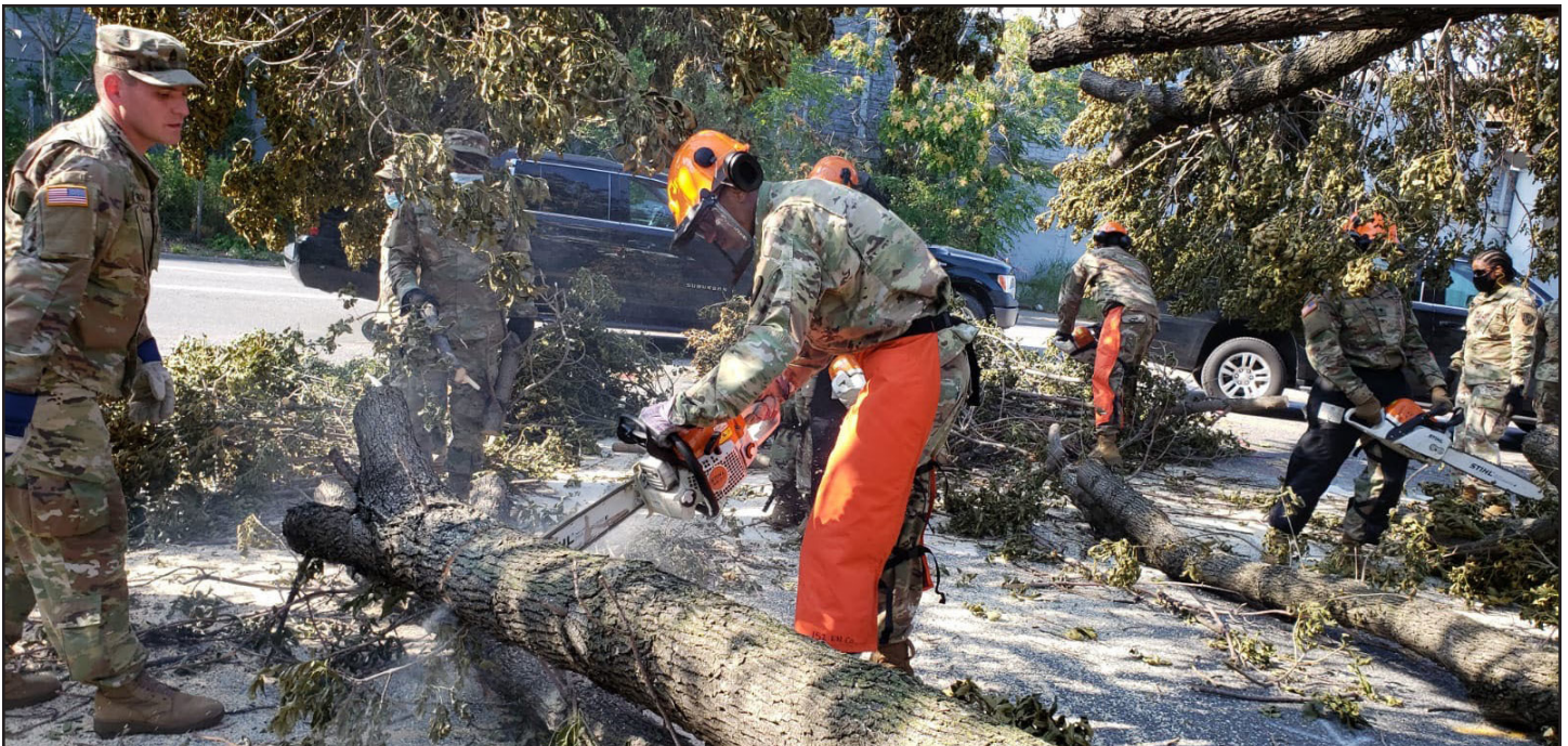
Soldiers and Airmen assigned to Joint Task Force Empire Shield, the New York National Guard's State Active Duty security force in New York City, clear downed trees at near the intersections of the Queens Midtown Expressway and 71st Street in Maspeth, New York on August 8, 2020. Courtesy photo.
