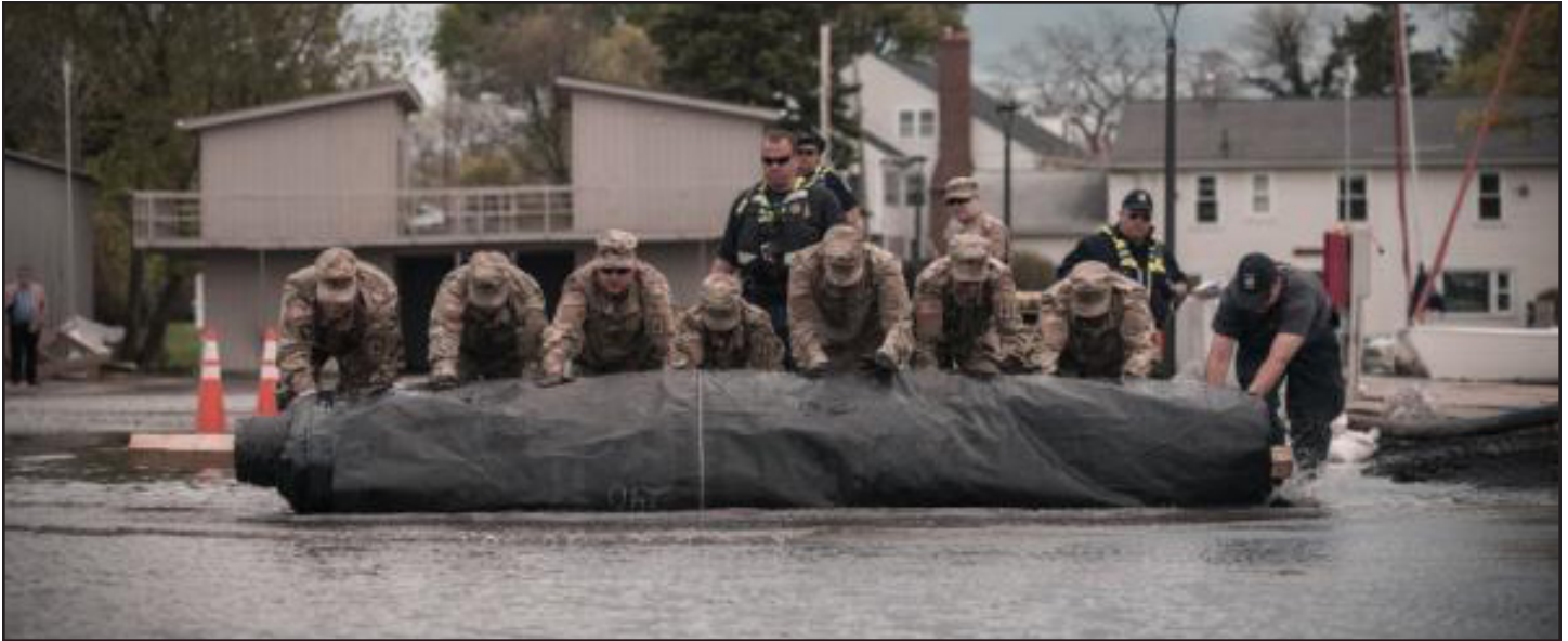
Soldiers assigned to the New York National Guard roll out a water-filled dam through flooded areas of the Port of Rochester, May 20, 2019. Gov. Andrew Cuomo activated the New York National Guard and Naval Militia after water levels in Lake Ontario started rising and causing flooding across areas of New York State. Photo by Ryan Campbell, Guard Times Staff.
