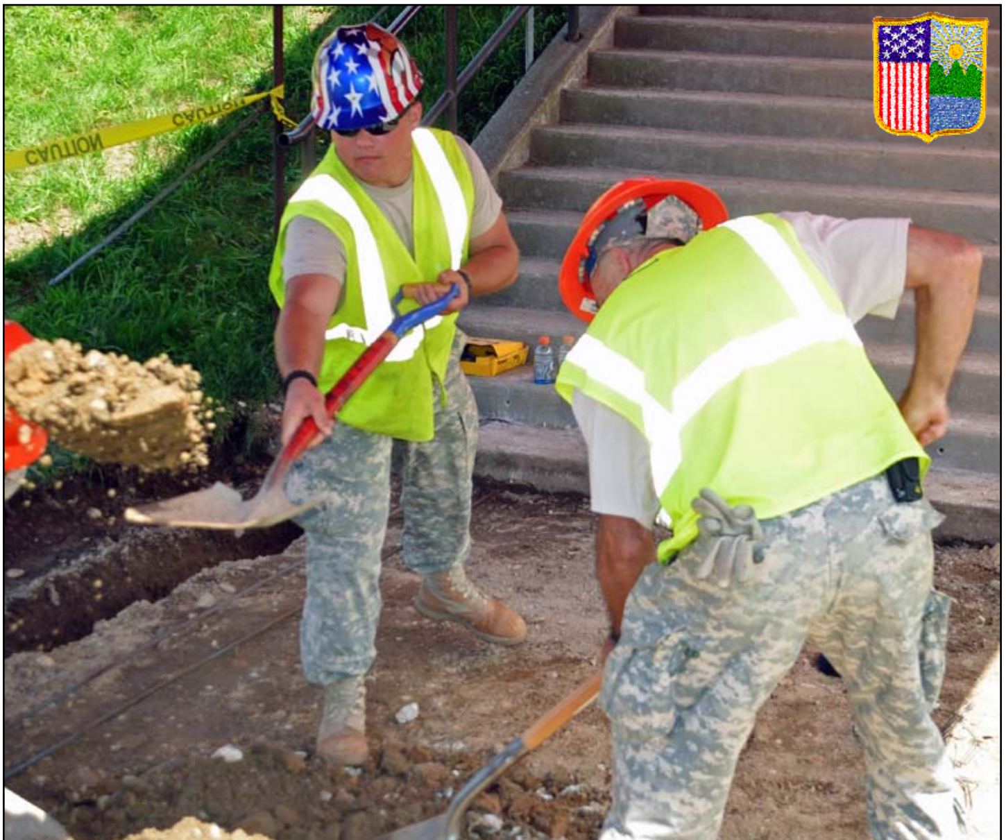
During their annual training in August, New York Guard troops level an area in front of Baker Hall so concrete can be poured. The work was one of the engineer projects New York Guard troops performed to improve Camp Smith. Photo by Capt. Mark Getman, New York Guard.
