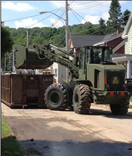
Engineers and Military Police Soldiers work together to help with debris clearance in Mohawk, N.Y. on July 3. Photo by Lt. Col. Christopher Panzer, Joint Force Headquarters.
