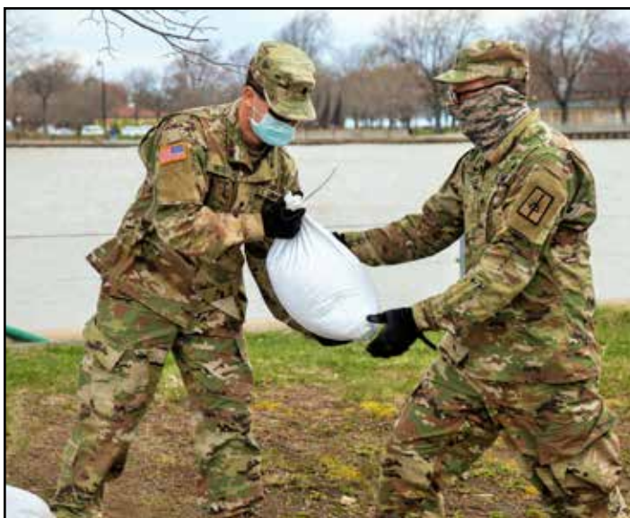
Soldiers assigned to JTF Ontario build a sandbag wall in Rochester near the Monroe County Sheriff Boat Launch on April 29, 2020. New York mobilized 46 members of the New York Army National Guard, the Naval Militia and New York Guard to respond to flooding along the Lake Ontario shore line. Photo by New York Guard Officer Candidate Michael Rehbaum.
