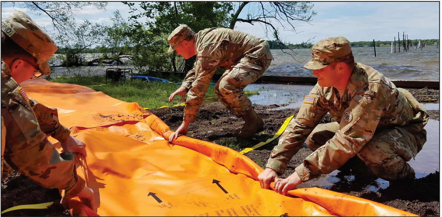
New York Army National Guard Soldiers deploy the Tiger Dam flood control system along the shores of Braddock Bay in the Town of Greece, N.Y. in response to rising waters on Lake Ontario. The system consists of flexible fabric tubes which are connected and filled with water. The tubes replace sandbags as a flood control mechanism. Photo by Sgt. Lucian McCarty, Joint Force Headquarters.
