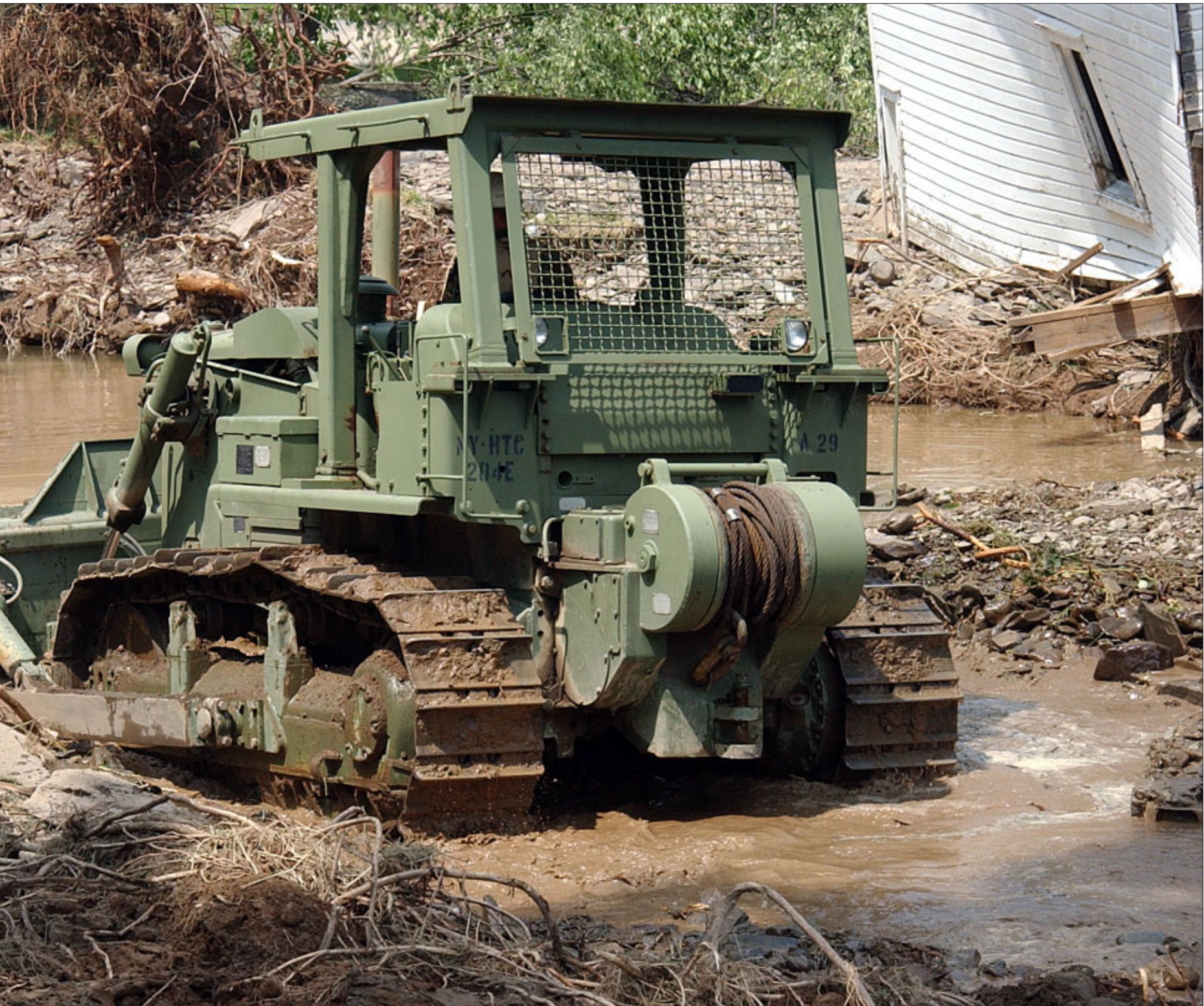
's 204 th Engineer Battalion moves debris in an effort to block a corner of a retaining wall that was washed out during the flood in Walton. Photo by Sgt. Ed Balaban.
