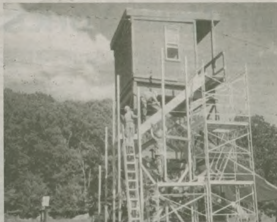
Engineers from the NY Guard's 102d Battalion conduct project improvements to the US Military Academy at West Point, NY. The construction, part of the unit's Annual Training, provided construction of buildings for Military Operations in Urban Terrain (MOUT) and construction of new stairs to the range control tower on the Tube-Launched Optically-Tracked Wire-Guided (TOW) Missile range. The range improvements will benefit West Point Cadets as well as Reserve and National Guard members who routinely use the Military Academy training areas and ranges for weapons qualification training. Photos courtesy of the NY Guard.
