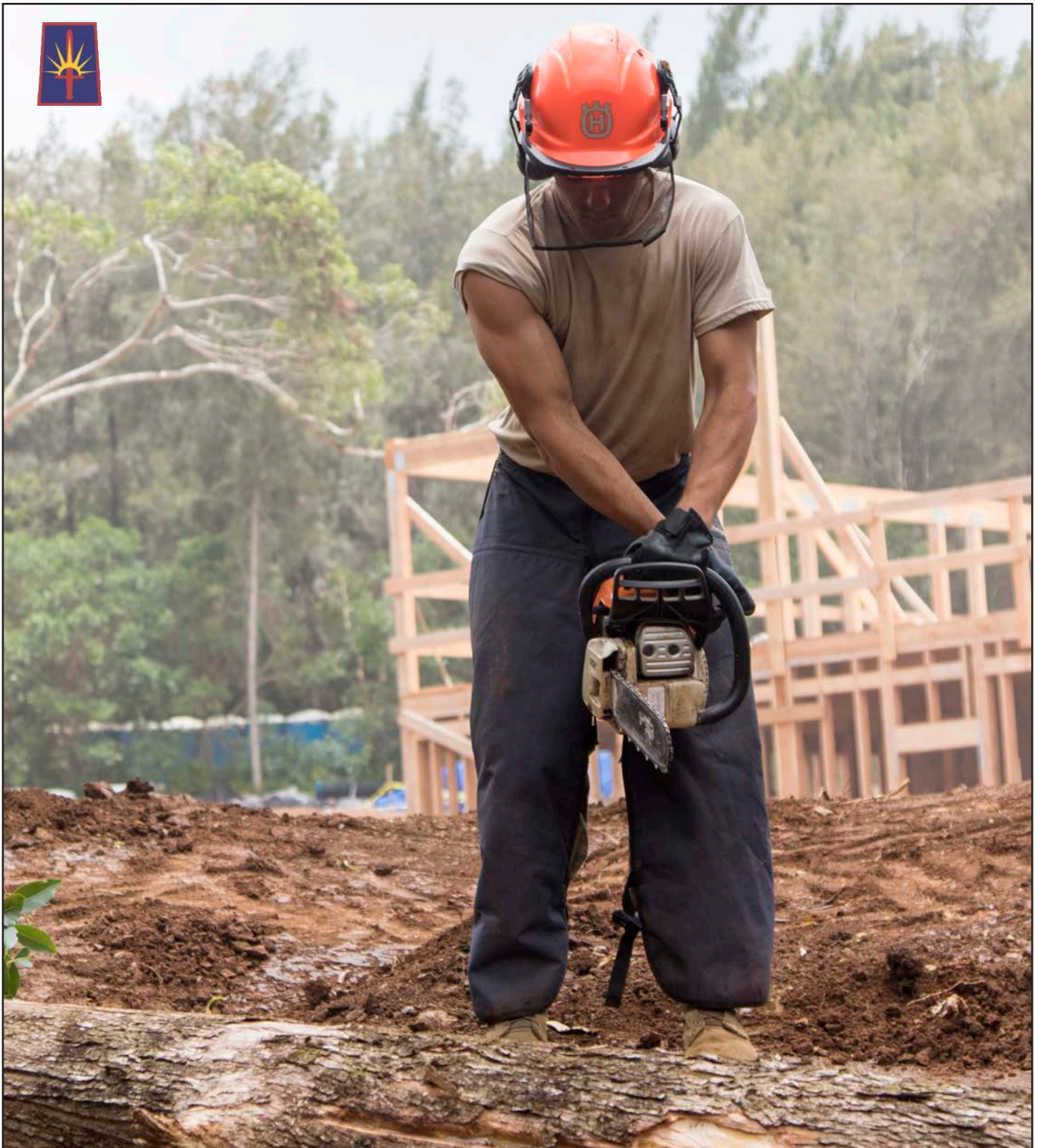
Pfc. Anthony Allen, a carpentry and masonry specialist assigned to the 1156th Engineer Company, 204th Engineer Battalion, operates a chainsaw to cut a downed tree into removeable sections during Innovative Readiness Training (IRT) at Girl Scout Camp Paumalu in Haleiwa, Hawaii, July 31, 2019. The Engineers joined other Air Force, Air National Guard and Marine Corps personnel since May to build a Science, Technology, Engineering, and Math activity center.
