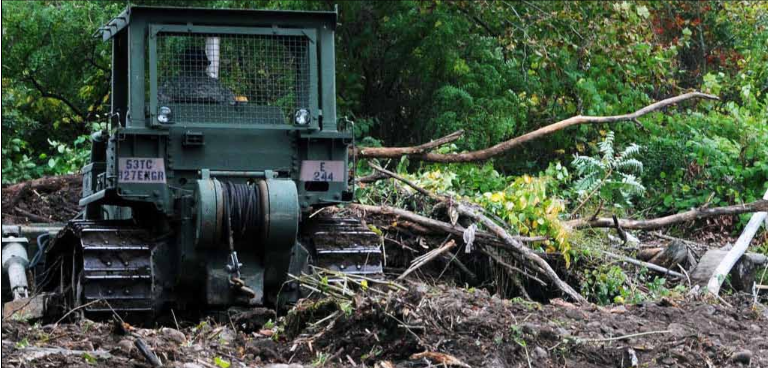
Soldiers with the 827th Engineer Company remove debris from the Esopus Creek in preparation for Hurricane Joaquin, Oct. 2. Photo by Sgt. Michael Davis, 138th Public Affairs Detachment.
