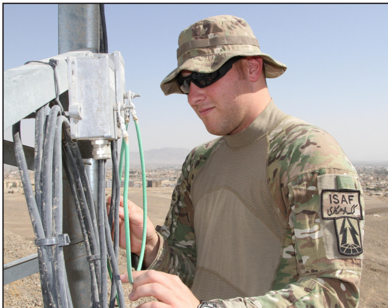
Senior Airman Matthew Perry, an engineer in the 213th Engineering Installation Squadron, 105th Airlift Wing, inspects wires at the base of a communications tower.
