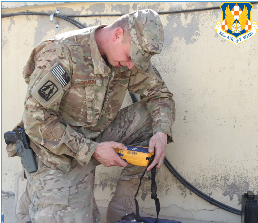
Capt. Michael Gielbeda serves as a cyber operations officer and the project engineer of communications for Regional Command South at Kandahar Airfield, Afghanistan. Gielbeda is with the 105th Airlift Wing's 213th Engineering Installation Squadron, based at Stewart Air National Guard Base in Newburgh. Photo by Cpl. Clay Beyersdorfer, 70th Mobile Public Affairs Detachment.
