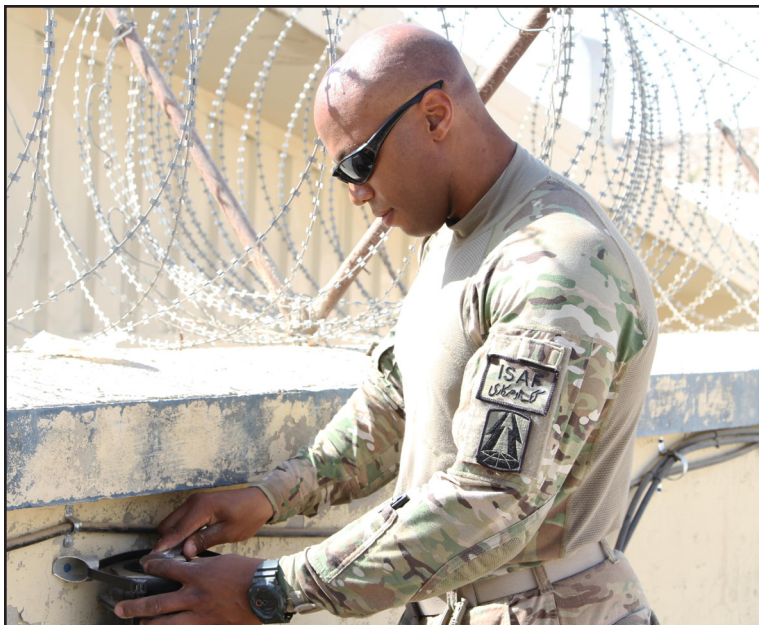
Staff Sgt. Greg Depass, an engineer in the 213th Engineering Installation Squadron, inspects an electrical box for faults or damage.
