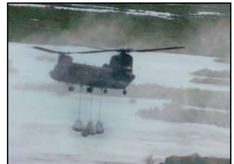
New York Army aviation Soldiers use their Chinook to build a levee during Hurricane Gustav
